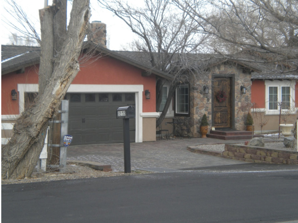
Garage, looking west from Valley Springs Road
