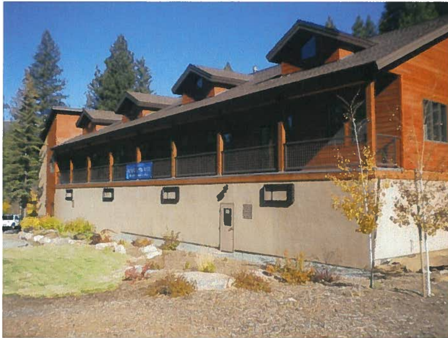
Front of Existing Building
