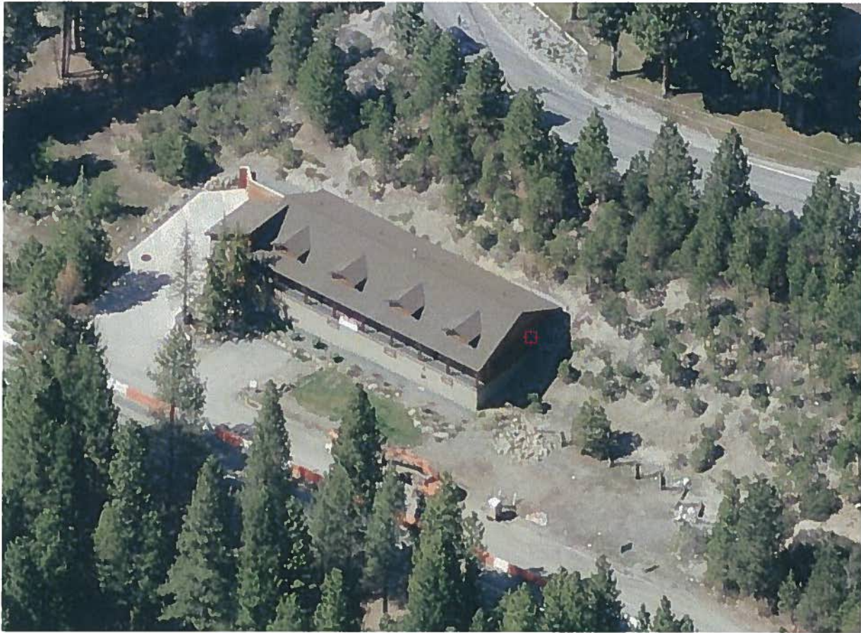
Overhead View of Existing Building
